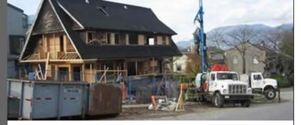
Recently, Sonic Drilling Ltd. was contracted to install four geothermal holes and loops for an older heritage-style home. The home was located on a difficult slope, with tight consolidated material underneath and in the middle of Kitsilano, a popular but congested urban neighbourhood in Vancouver, BC.
